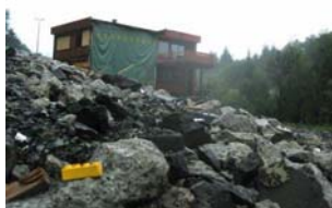
Heavy rainfall contributed to the Hatlestad mud and rock slide in Norway in 2005.
